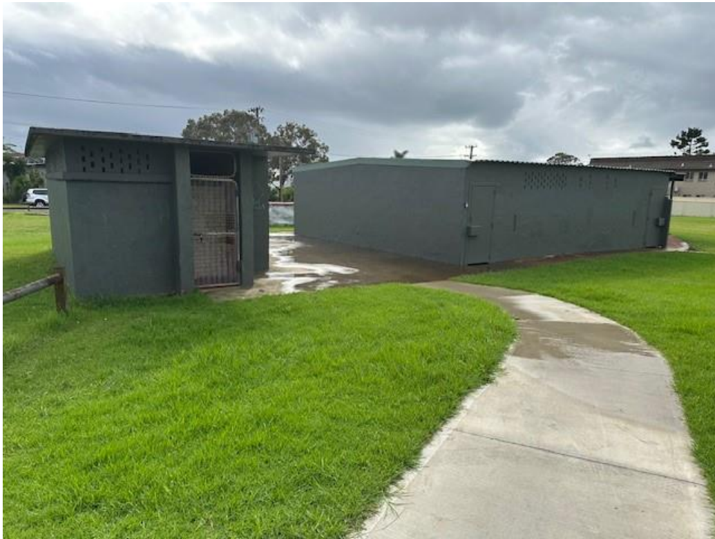
Figure 3 – Existing sport club house
