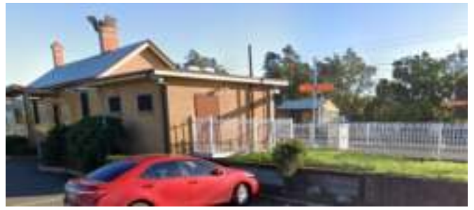
▲ Albion Park Station
