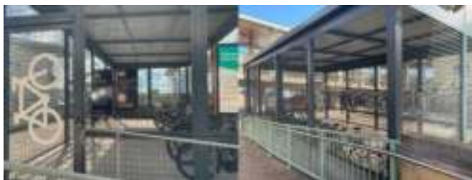
▲ TfNSW bicycle shed, Hornsby Station
