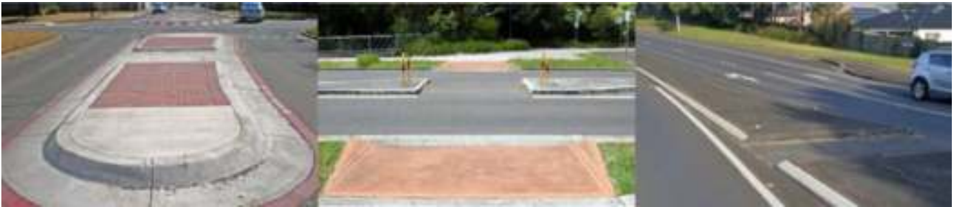
▲ Median, pedestrian refuge and splitter island
