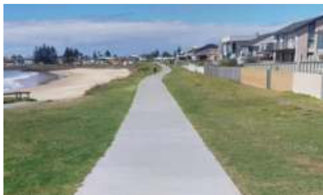
▲ Narrow shared path from Bucknell Street to Elliott Lake Bridge
