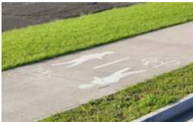
▲ Shared path markings, Junction Road
