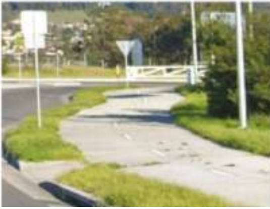
▲ Delineated right of way (Croome Road, Croom)
