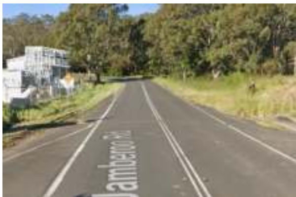
▲ Jamberoo Road aerial shot and road perspective
