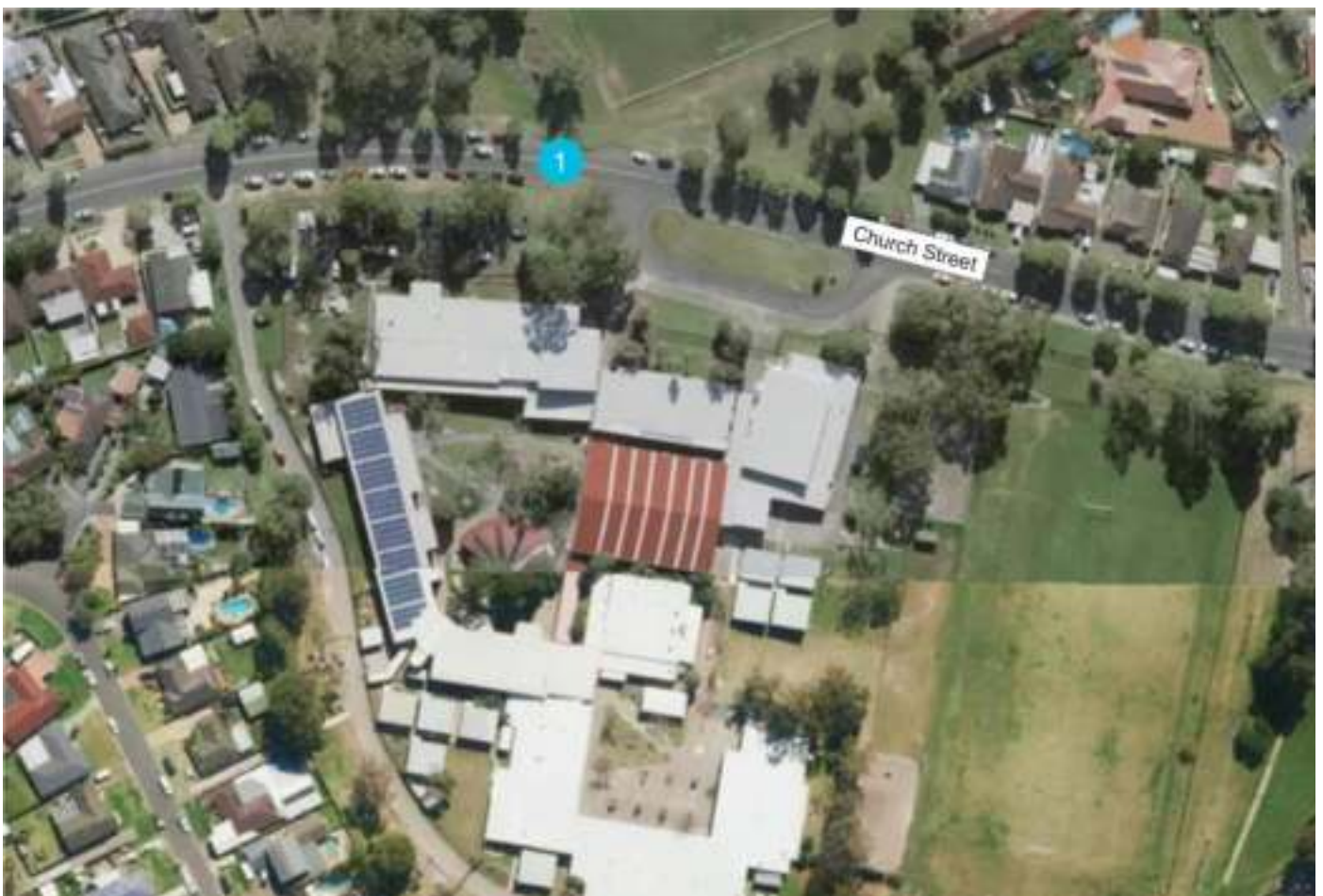
▲ Albion Park High School location of safety improvement measures
