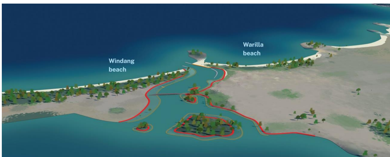
Above: The Lake Illawarra entrance channel showing foreshore areas subject to erosion
