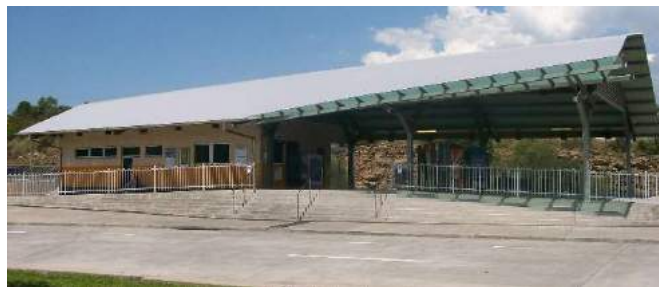
▲ Oak Flats Station
