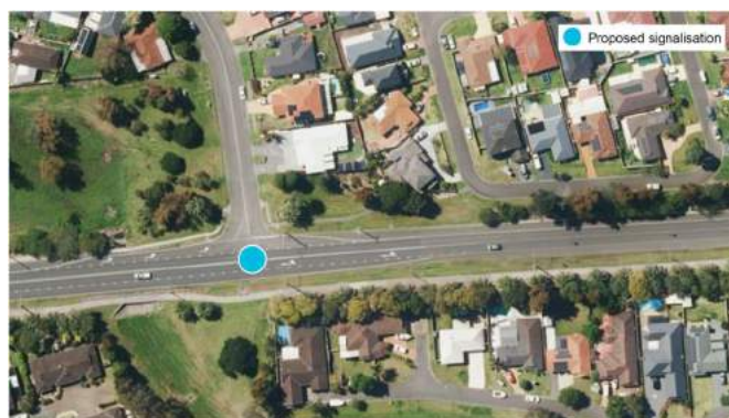
▲ Location of upgrade to signalisation at Terry Street / Burdekin Drive intersection
