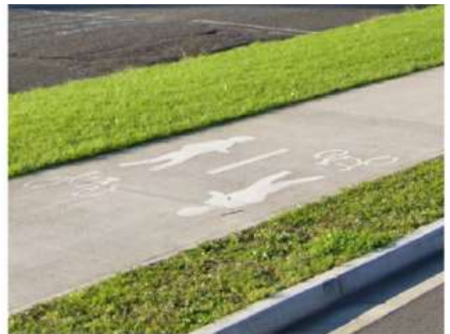
Regular path markings (Junction Road, Shellharbour)
