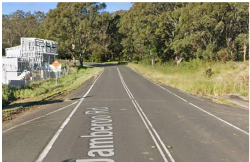
▲ Jamberoo Road aerial shot and road perspective
