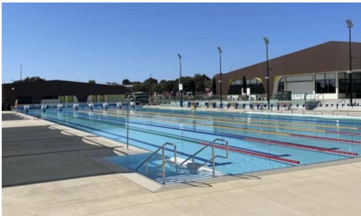
Figure 75 – North Bellarine Aquatic Centre
