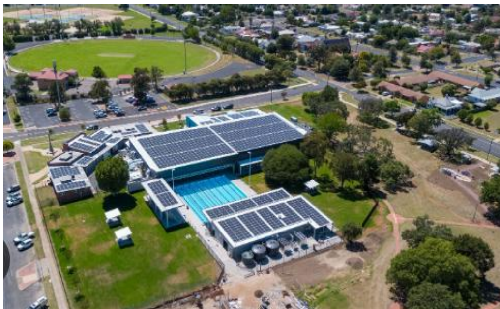
Figure 76 – Inverell Aquatic Centre
