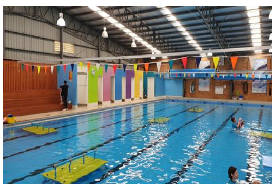
Shellharbour Swim Academy heated indoor 25m pool
