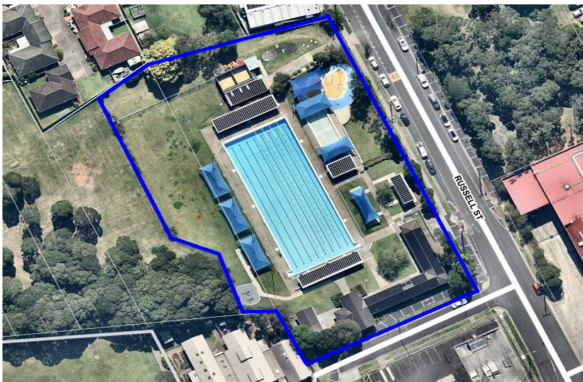
Figure 13 – Overview of Albion Park Pool Site
