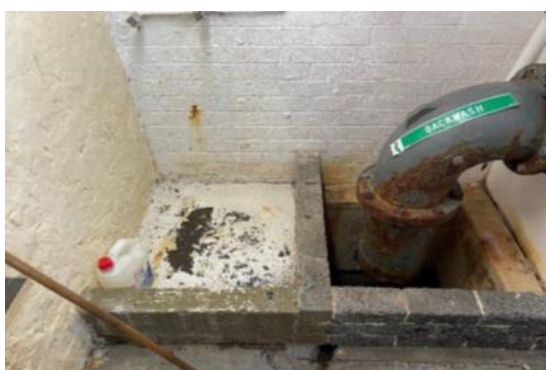
Warilla Pool backwash outlet pipe and sump
