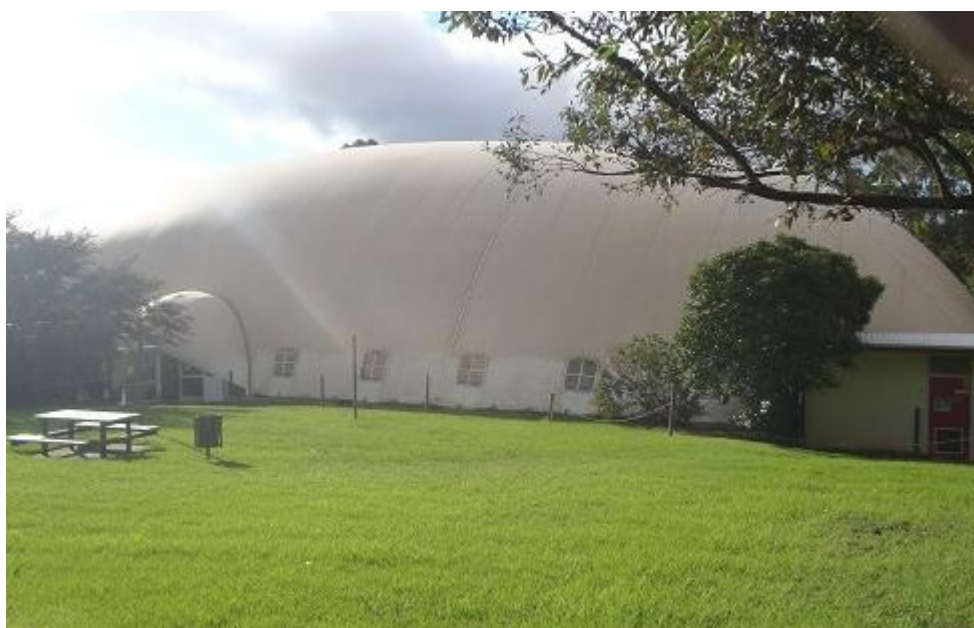
Figure 74 – Kilsyth Centenary Pool
