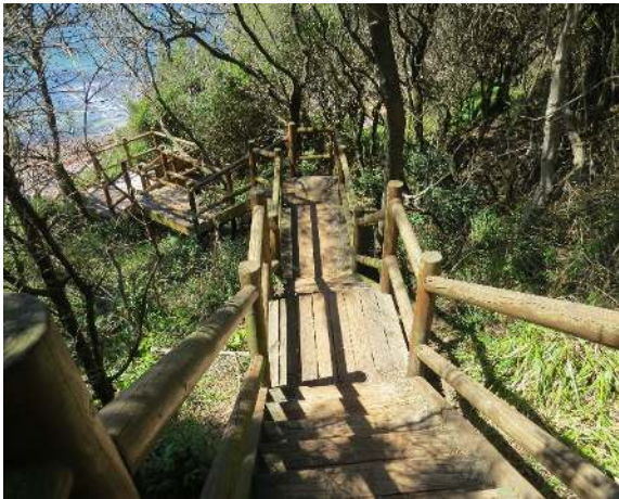
Figure 5: Stair access at Bushrangers Bay
